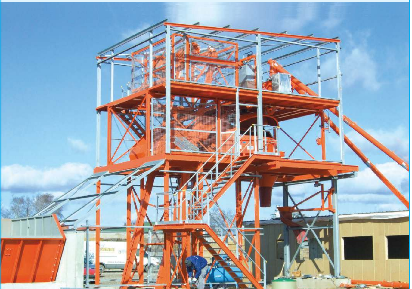
Montage MIXOMAT THZ 3000 - R 4 / 4 Reihen-Siloanlage, 4 Kammern • Erection MIXOMAT THZ 3000 B - R 4 / 4 aggregate in-line silo system, 4 compartments
