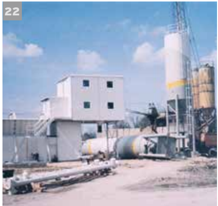
18-22 | Erection of MIXOMAT THZ 3000 C 1-R with heavy duty TEKA pan-type mixer with separate mixer and weighing scale platforms and complete housing for the plant.
