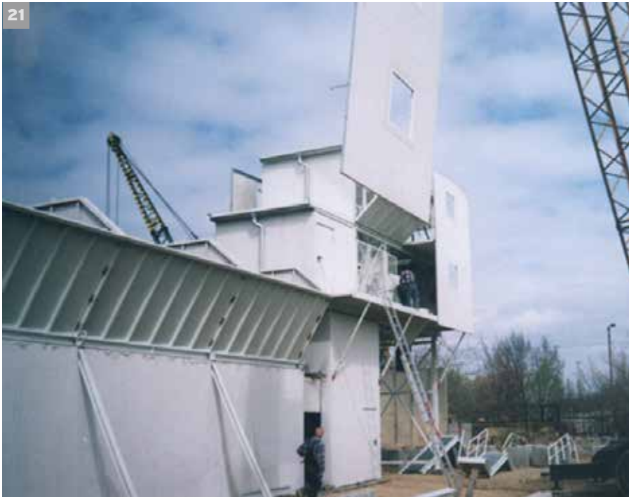
18-22 | Erection of MIXOMAT THZ 3000 C 1-R with heavy duty TEKA pan-type mixer with separate mixer and weighing scale platforms and complete housing for the plant.
