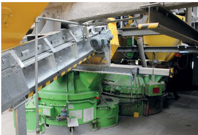
General view of the mixer level: Teka THT high-performance turbine mixer for the facing concrete and Teka TPZ 1125 planetary mixers for the core concrete
