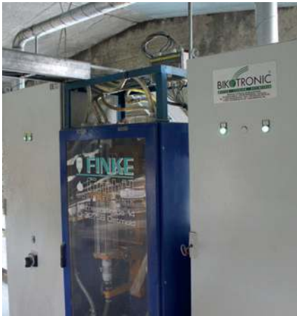
The admixtures are metered by the Finke system with visually inspectable weighing hopper in the dustproof cabinet.
