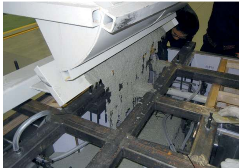
Concreting the first component
