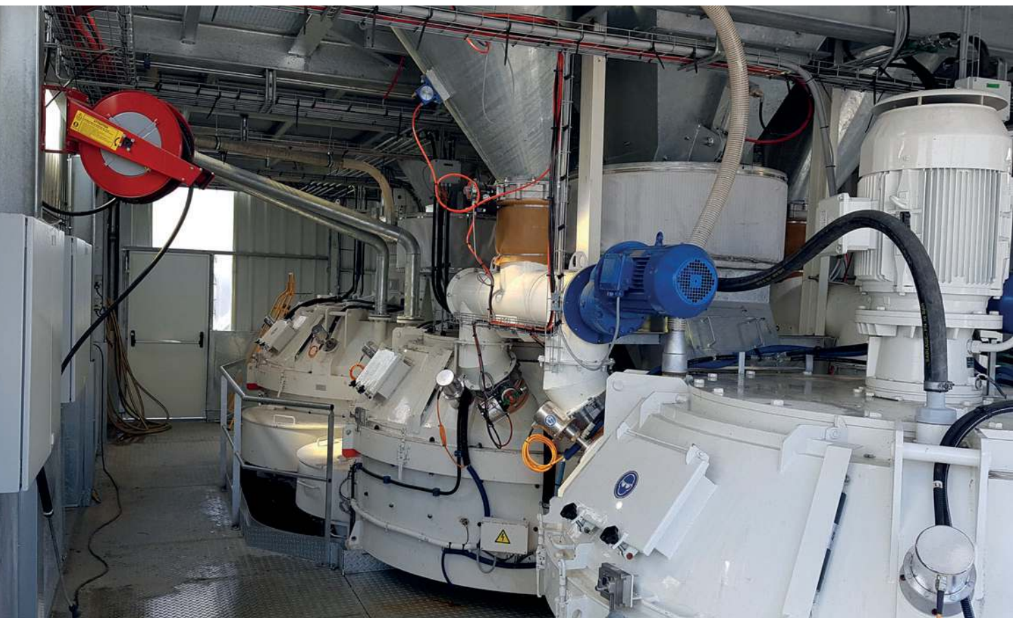
The new mixing plant has 3 Teka mixers, each equipped with an automatic high-pressure cleaning system.
