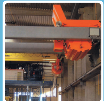
Rollover bucket and concrete distributor
