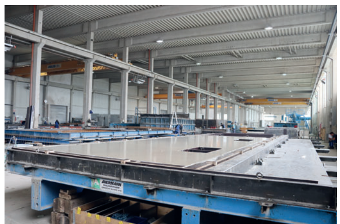
The circulation system for ceiling and double wall production was supplied by Avermann at the time.
