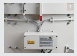
7 | Electrical components are completely pre-wired to an electrical junction box.
